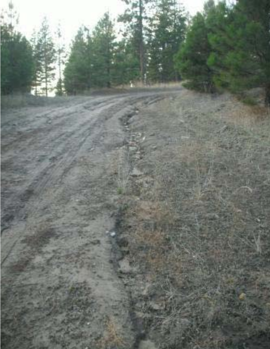
Photo 11: Minor rill erosion in existing unimproved road, west side of proposed project facility location.
