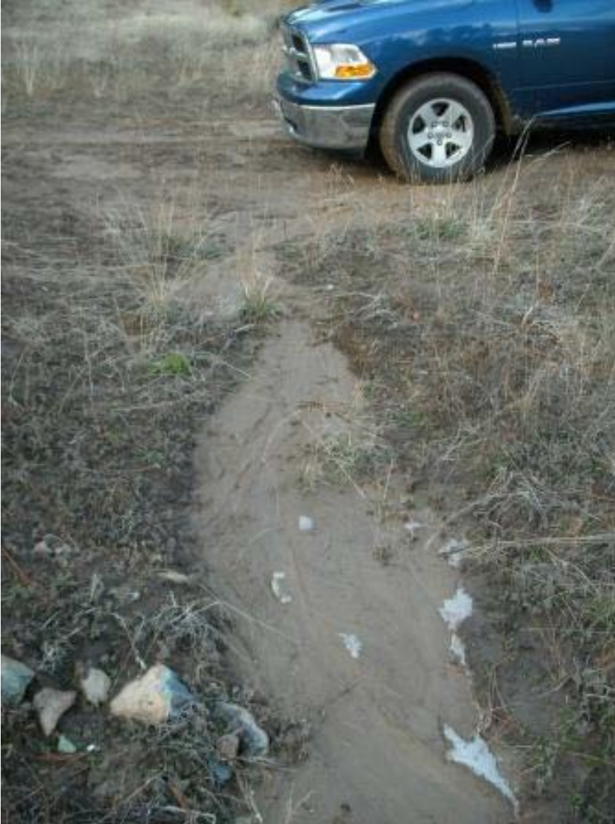
Photo 12: Sediment transport at low road crossing on unimproved road.
