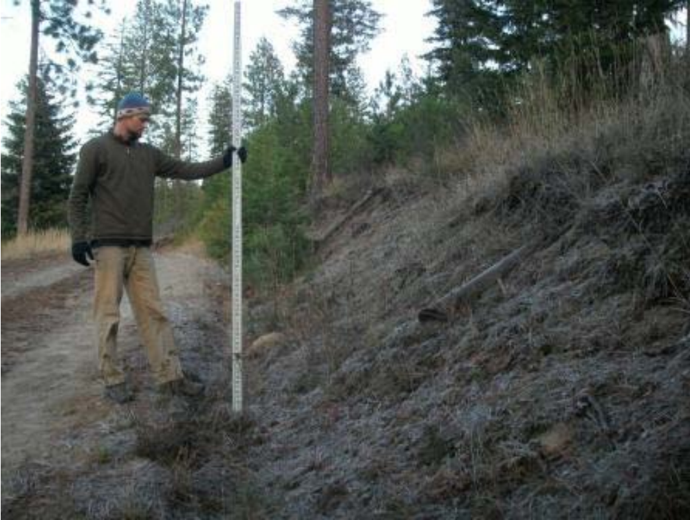
Photo 7: Road cut between east and west portions of proposed project facility location. Note lack of erosion and stable cut slope.
